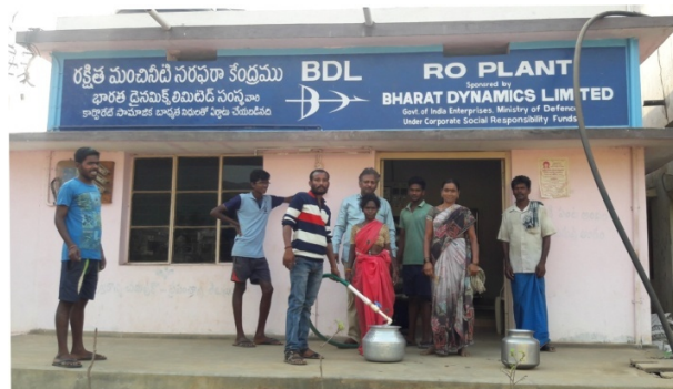
BDL newly installed an R.O Plant at Gondupalem Village, K.KotapaduManal, Visakhapatnam District, Andhra Pradesh
