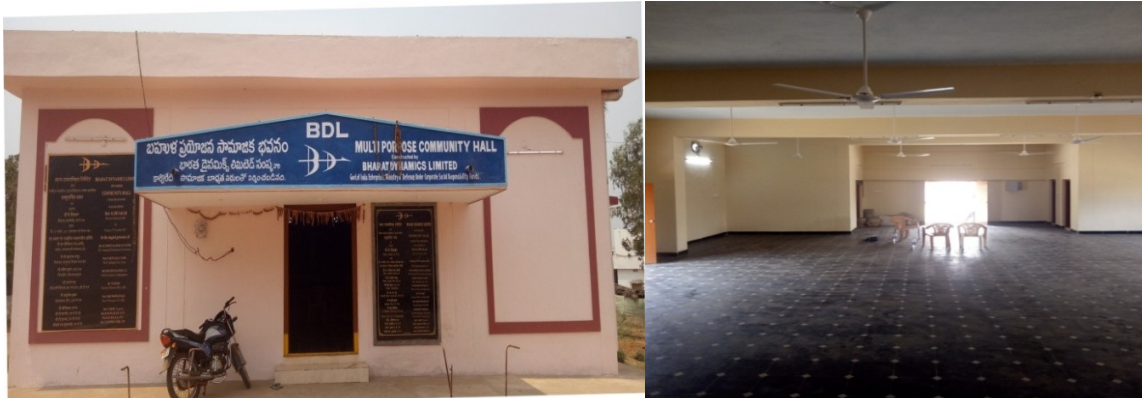
BDL Newly Constructed Community Hall at Gondupalem Village
