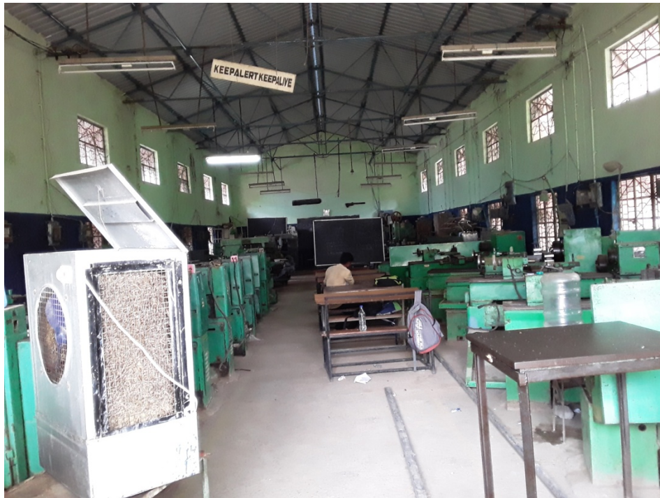
Renovation of workshop by removing of Asbestos sheet and laying new Galvanized Sheet
