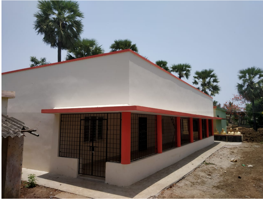
BDL Constructed 2 class rooms in Primary School, Madhavaram under its Village Adoption Program
