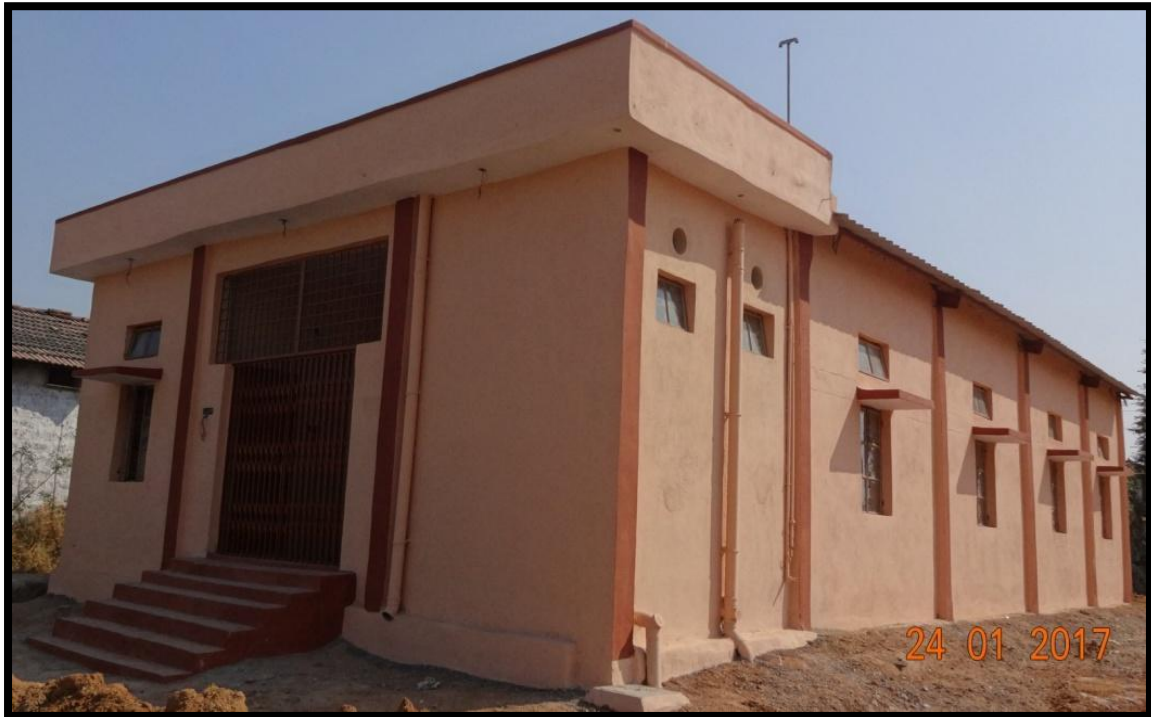
NEWLY BUILT COMMUNITY HALL AT KYSARAM VILLAGE, MEDAK DISTRICT, TELANGANA STATE
