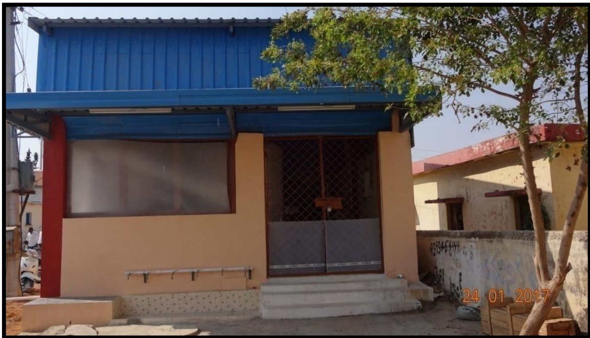
NEWLY BUILT RO WATER TREATMENT PLANT AT KYSARAM VILLAGE, MEDAK DISTRICT, TELANGANA STATE
