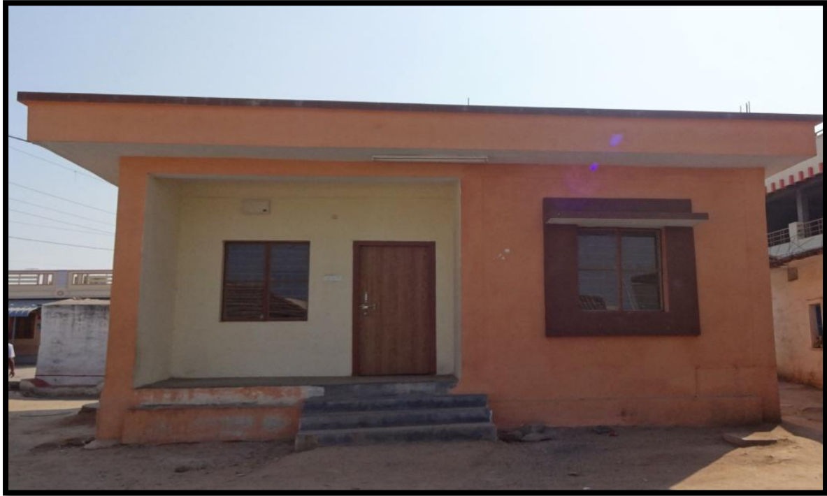
NEWLY BUILT PRIMARY HEALTH CENTRE AT KYSARAM VILLAGE, MEDAK DISTRICT, TELANGANA STATE
