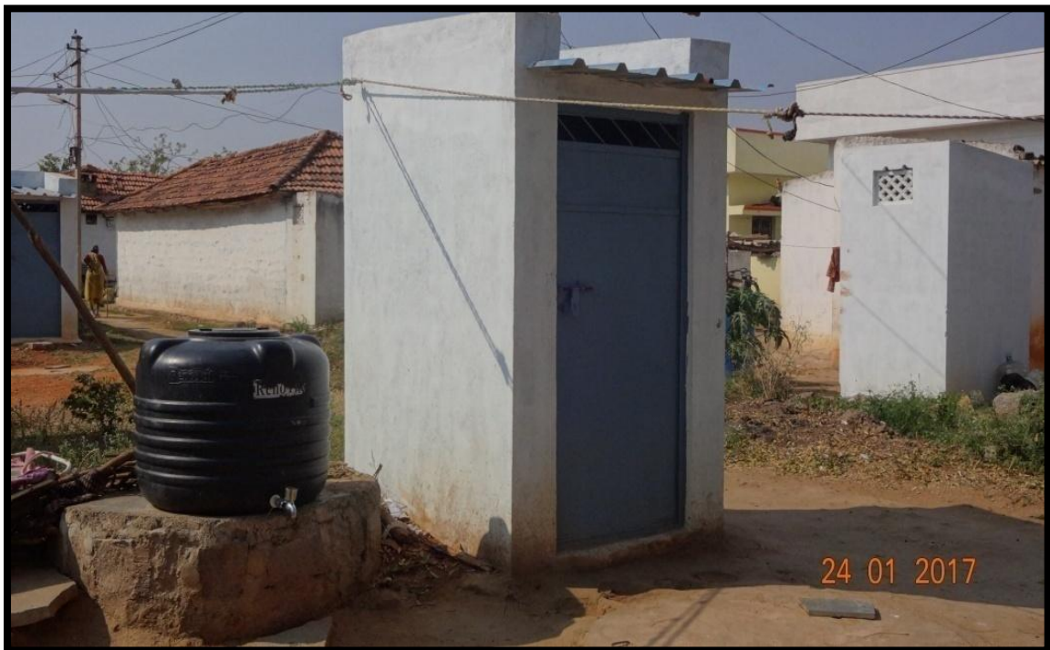
BDL CONSTRUCTED INDIVIDUAL HOUSEHOLD TOILET BLOCKS AT KYSARAM VILLAGE, MEDAK DISTRICT, TELANGANA STATE
