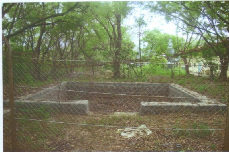
5m X 5m Rain Harvesting Pit behind transport (Corner of EP shop)
