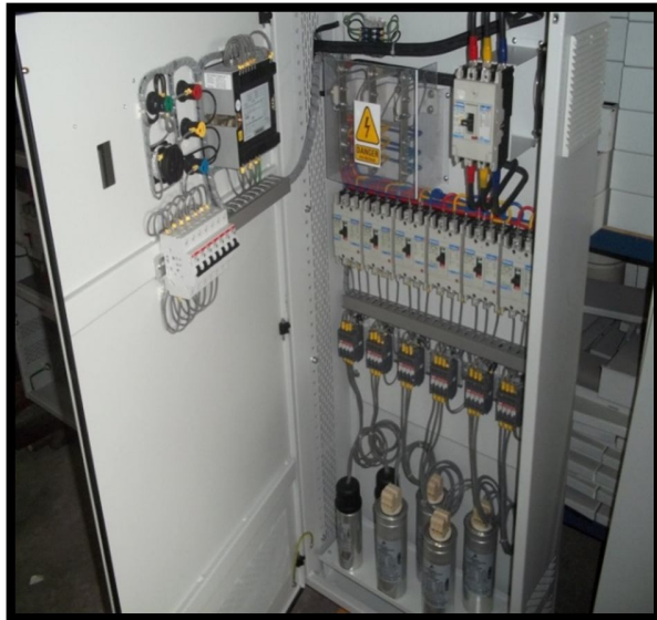
Automatic Power factor Control panel (Typical)
