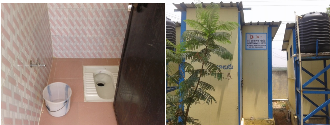
Maintenance of school toilets at M.P.P.S school Marripally, Hayathnagar Mandal, Rangareddy District.
