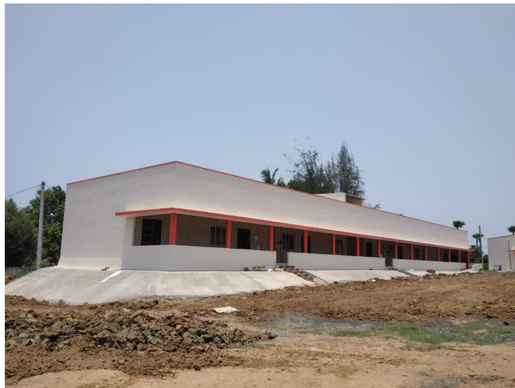
BDL Constructed new class rooms in ZPHS High School, Madhavaram under its village adoption programme
