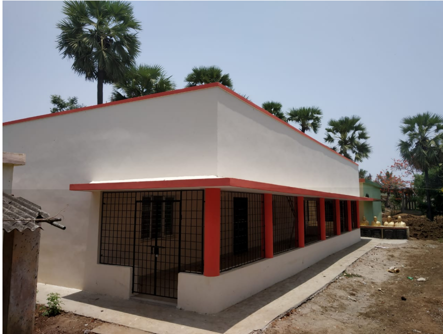
BDL Constructed 2 class rooms in Primary School, Madhavaram under its Village Adoption Program
